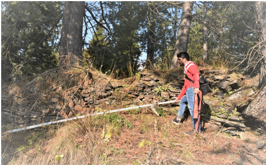
Fig.3. Masonry rubble wall at Khimar Pathri (Photo: Yasir)
